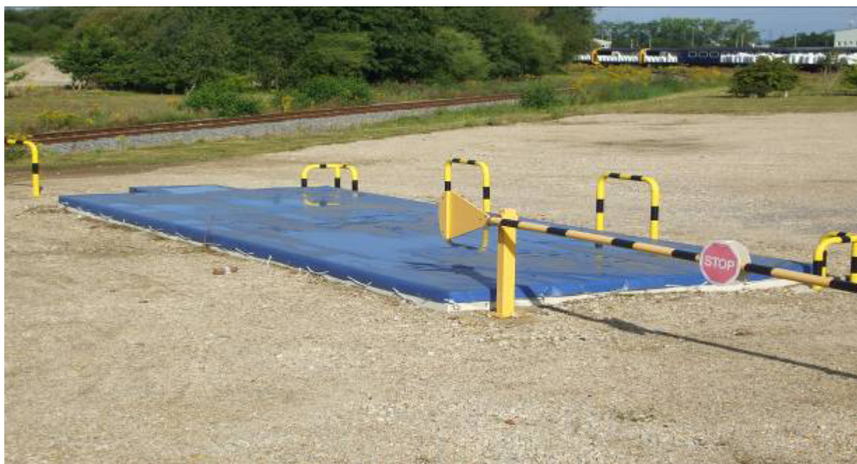
The above container bund is located near the waterfront adjacent to the container section/weighbridge
