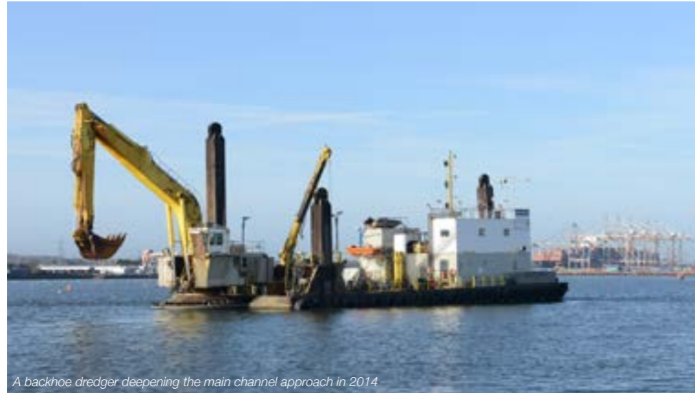
A backhoe dredger deepening the main channel approach in 2014
